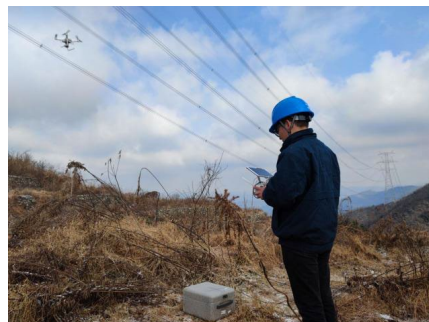
Figure 1. Workers Carry Out Inspection of Ultra-High Voltage Lines.
